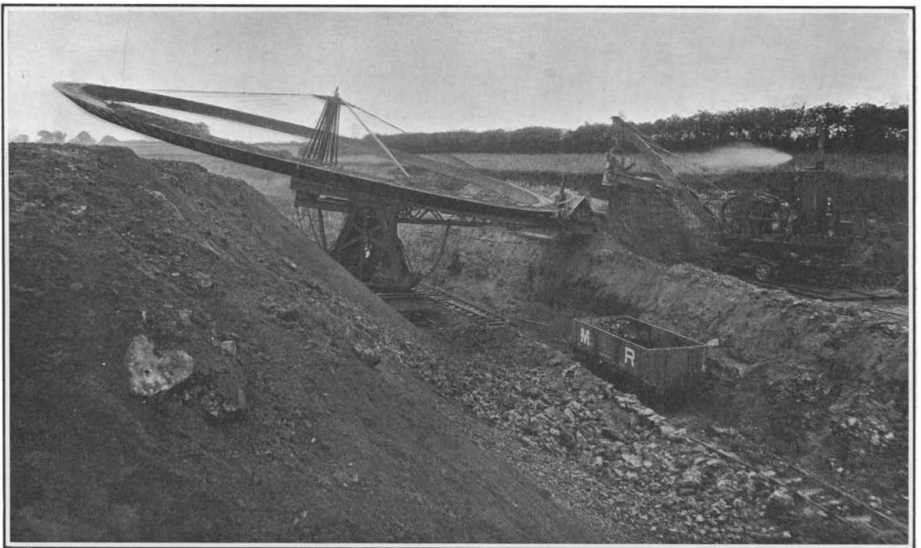
Side view of the rotary conveyer. The conveyer is traveling from the observer.
