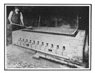
**Oven in which the damascening is done.** The articles to be decorated are covered with metal dust and then heated to the required temperature.
