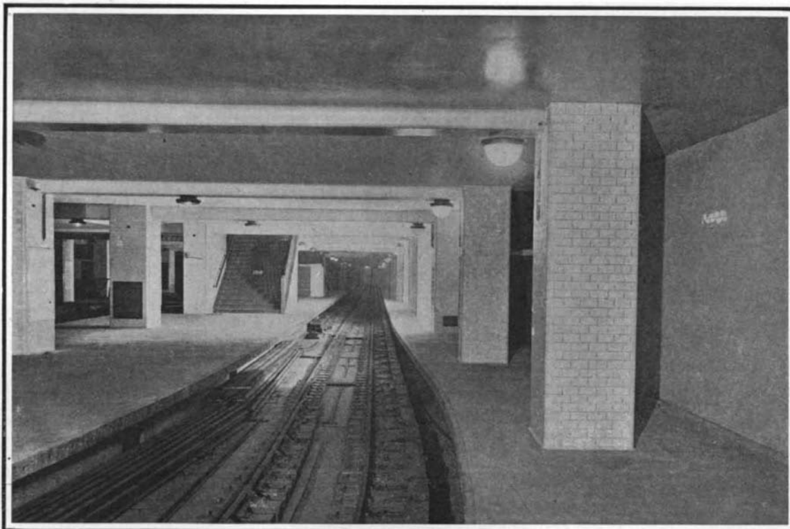
TRAIN LEVEL AT HUDSON TERMINAL, LOOKING NORTH ON WEST SIDE.
