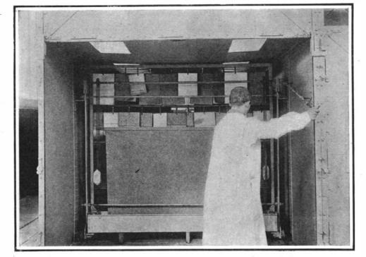
Fig. 4.-Agitating the felt saturated with formic aldehyde.
