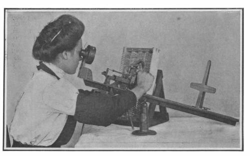
Centering the lens. This operation is highly important; for on the ink spot placed on the center of the lens depend the mechanical and optical properties of the finished lens.
