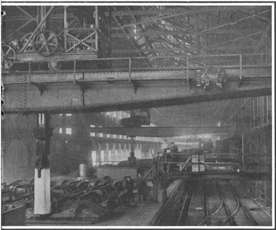
Here the ingots are heated in gas-fired underground furnaces to the proper temperature for rolling. The soaking pits.
