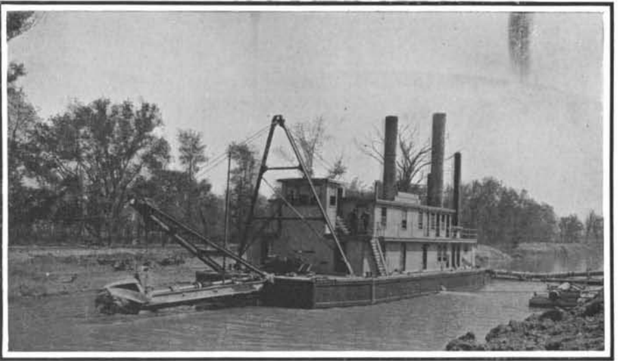
HYDRAULIC DREDGE EXCAVATING CHANNEL.
