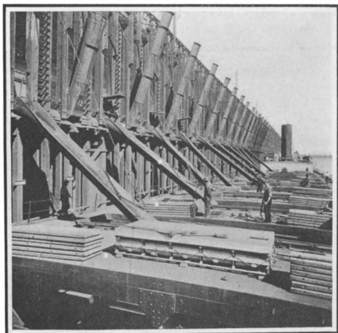
The ore discharges through spouts by gravity into the holds of the steamers.
