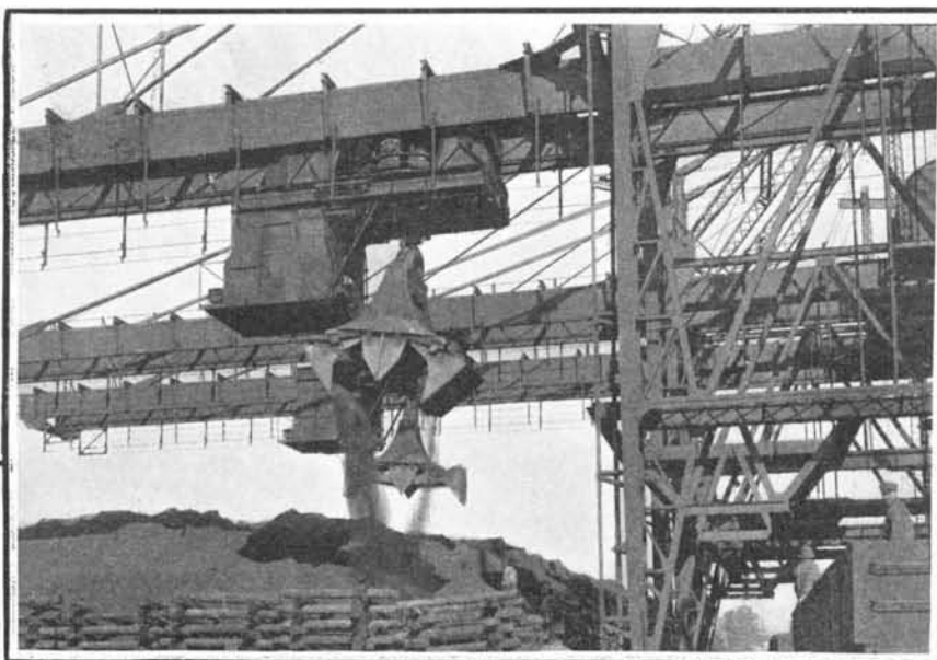
Five-ton buckets unloading material at the stock pile.
