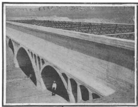
Concrete flume which carries inter-state canal across Spring Canyon.
