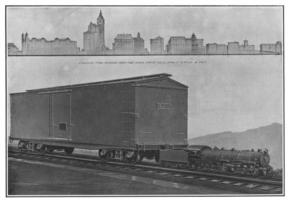
This huge Baldwin freight engine, weighing 300 tons, was built for the Southern Pacific Railroad. It is capable of hauling at 10 miles an hour a train of 169 cars weighing, with load, 72 tons each. The train, weighing 10,000 tons, would reach for over a mile or, say, from City Hall Square to the Battery, New York. The lower cut represents the size of a single car, 200 feet by 45½ feet by 62 feet, that would be necessary to contain the load of wheat handled.
