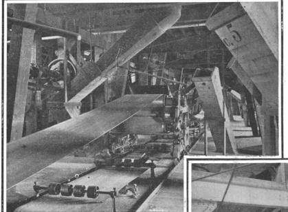
BELT CONVEYER AND TRIPPING MACHINES FOR DISCHARGING WHEAT FROM BELT.
