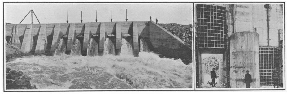
This view shows 22,000 second-feet passing through five 8 x 12 foot gates and five large and two small penstock openings in diversion channel. MINIDOKA PROJECT, IDAHO.
