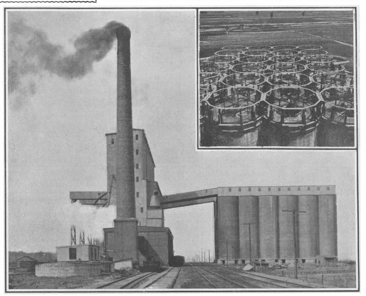
Upper view shows building of the concrete bins. The working house. SANTA FE ELEVATOR AT ARGENTINE, KANSAS. CAPACITY, 1,000,000 BUSHELS.
