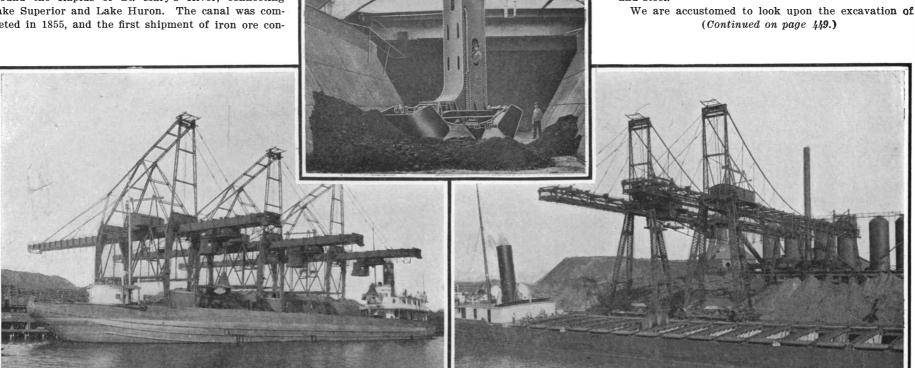
Length of bridge, 222 feet 8 inches. Bucket lifts 5 tons. THREE FAST PLANTS UNLOADING WHALEBACK STEAMER.
