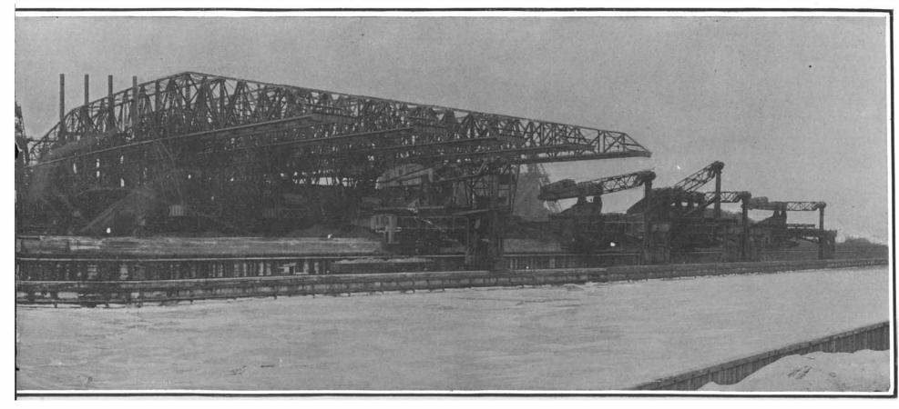
Five traveling conveyer bridges for transporting the ore to stock yard and furnaces.
