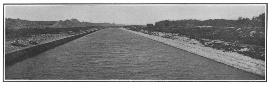
This great artificial channel, 22 feet deep, 110 to 202 feet wide, and 28 miles long, will form the first section of the Lakes-to-the Gulf waterway. MAIN CHANNEL OF DRAINAGE CANAL, ROMEO CURVE IN DISTANCE.
