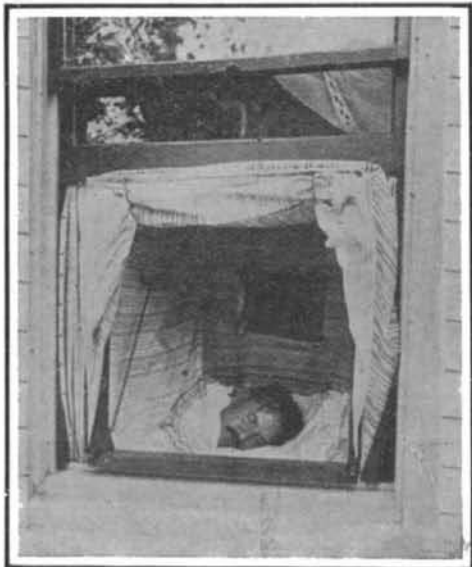
Storm awning raised, showing the sleeper in the indoor bed tent.
