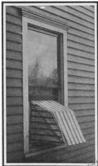
The storm awning outside the window.
