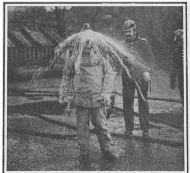
FIREMAN PROTECTED BY A SPRAY HELMET.
