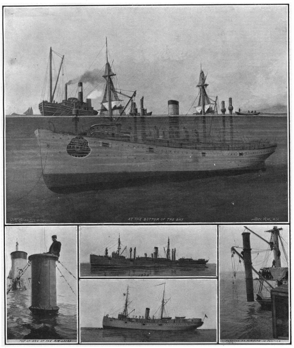
The old method of salvage was to close the rents in the hull and pump out the water. By the new method the ship is rid of water by forcing compressed air into the holds and displacing the water.
