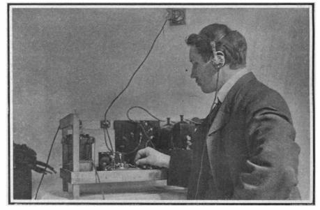
The wireless set employed by the Signal Corps for aeronautic usc. The total weight is about 70 lbs. An 8-volt, 20-lb. accumulator supplies the current.
