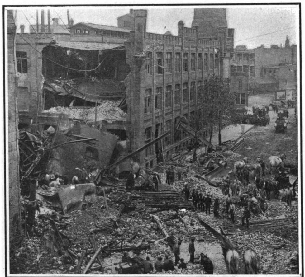
The debris covered this street to a depth of several feet. A large portion of the boiler was thrown across the street and landed on a roof of a 60-foot building.
