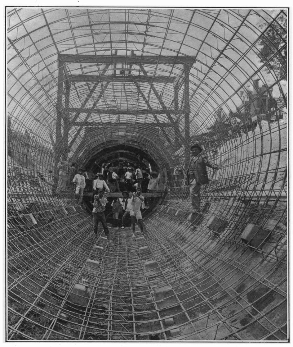
LOOKING THROUGH & REINFORCED CONCRETE CONDUIT IN COURSE OF CONSTRUCTION.-[See page 328.]
