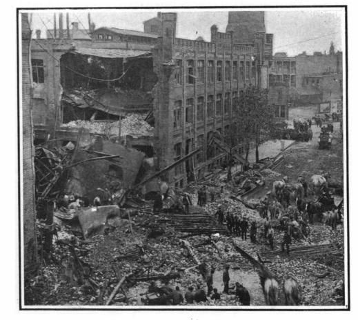
To the left is seen the wall of the building 60 feet high which was moved bodily a distance of 4 feet. The debris covered this street to a depth of several feet. A large portion of the boiler was thrown across the street and landed on a roof of a 60-foot building.
