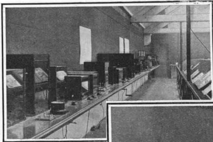
A row of static electrical machines.
