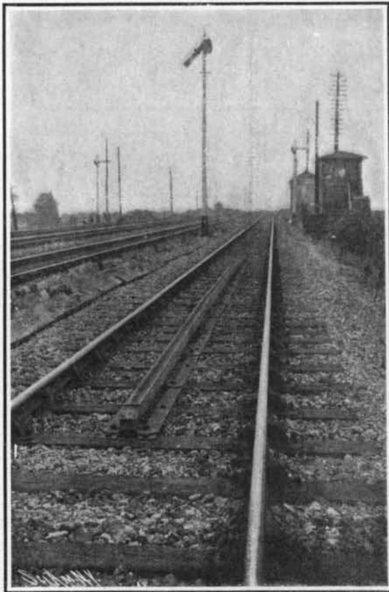
Section of track provided with central ramp.
