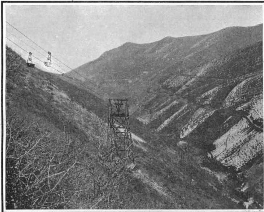
Aerial cable tramway sending down to the railway ores from the Utah Apex mine.
