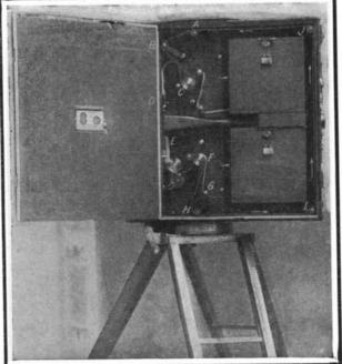
Showing system and mechanism for operating the endless band of color filters and how it is brought into juxtaposition with the sensitized film before exposure and separated therefrom after exposure.
