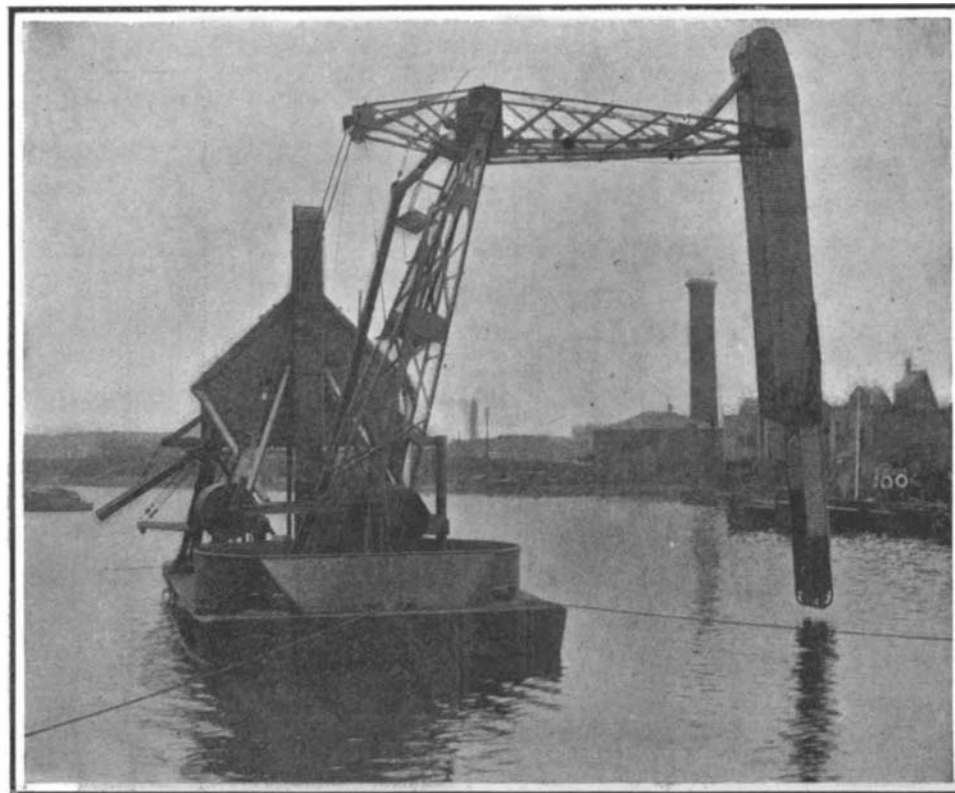
The elevator in mid-position as it would be when half way down into a ship's hold.
