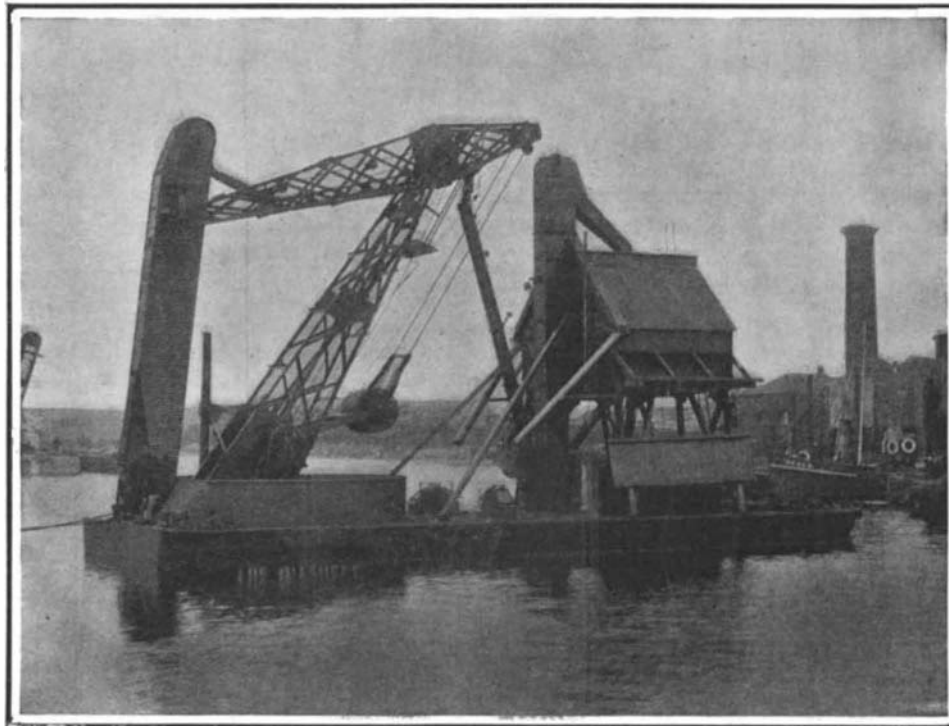
The elevator at rest upon the pontoon's deck for transit. This view well shows the parallel motion of cantilever arm and balance weight.
