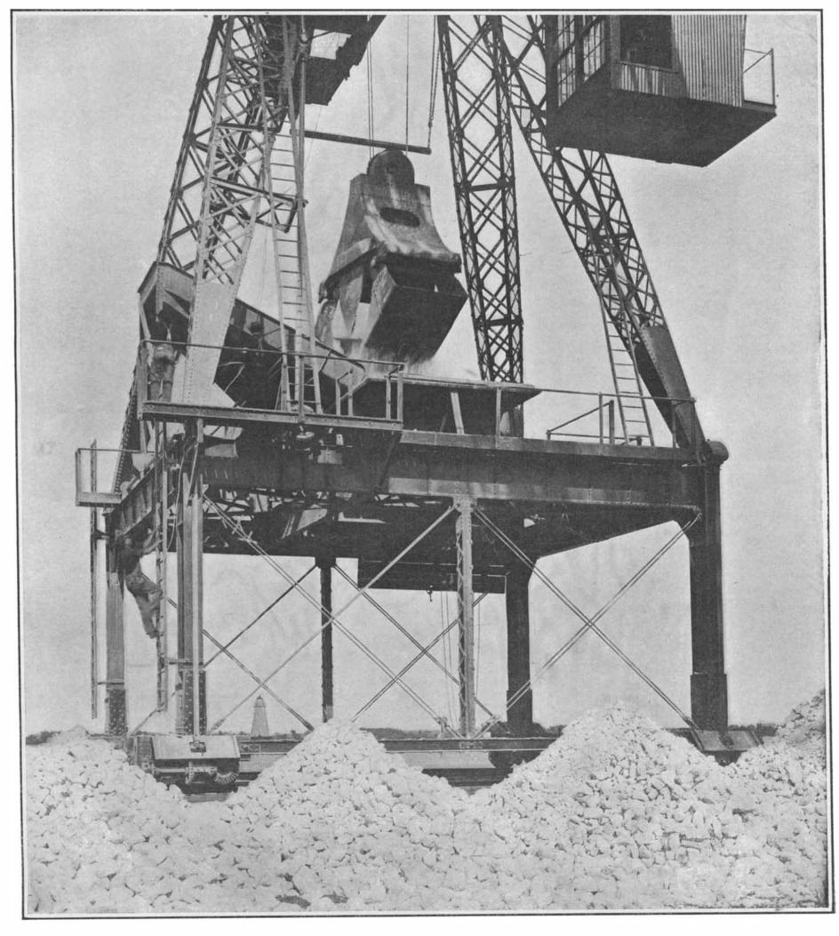
This machine can handle 200 tons of limestone per hour. The grab bucket, 7½ feet wide and 17½ feet long, when open can "grab" 100 cubic feet of limestone; hoist it at 275 feet per minute; and convey it to the desired position at a speed of 900 feet per minute.
