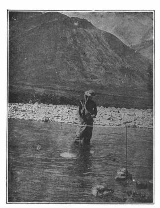
Gaging the flow of a mountain stream with hand instrument.
