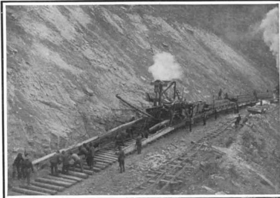
Laying track on the Chicago, Milwaukee & Puget Sound Railway.
