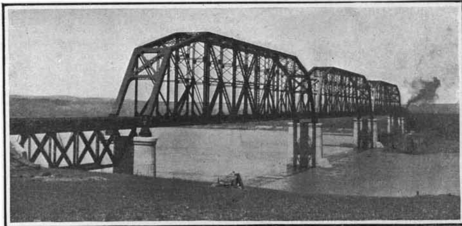
The three 423-foot spans of the Missouri River bridge.
