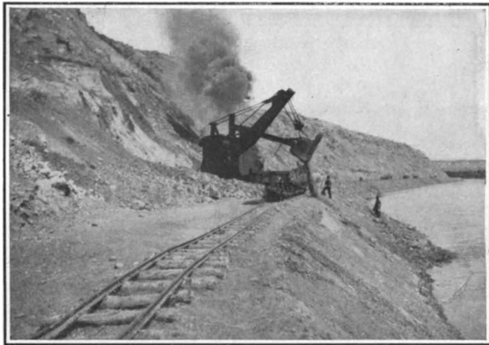
Steam shovel work at Lock Bluffs, Montana.
