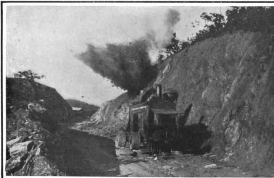
Between kilometer posts 10 and 18 on the Pinar del Rio-Luis Lazo road.
