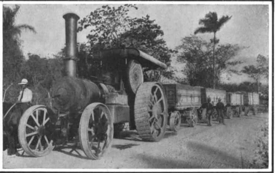
A traction train on an American-built road.
