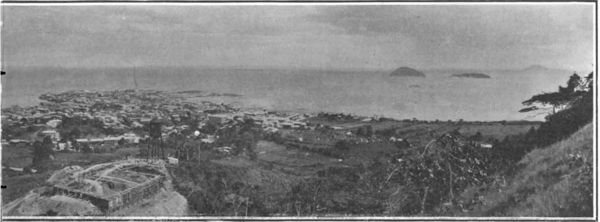
New concrete reservoir.
