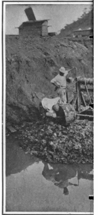
Test pit sunk to determine character below Miraflores dam
