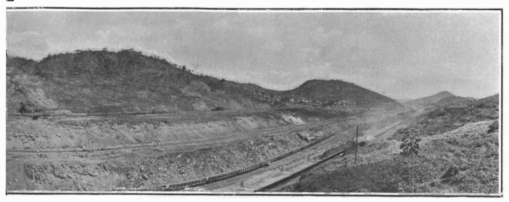
stretch between Gold Hill and Cucuracha is sliding, necessitating much extra excavation.
