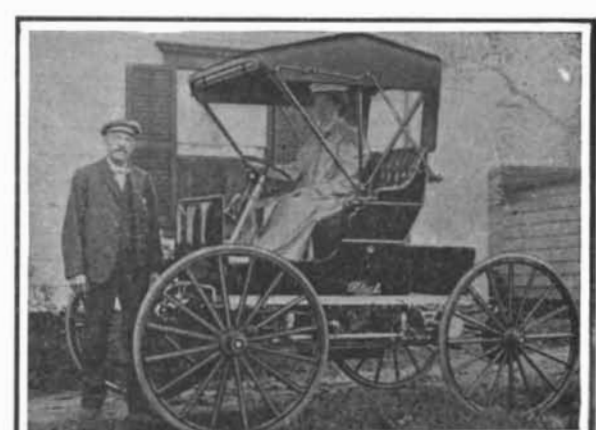
2-cylinder, 14-horse-power engine; planetary transmission; two speeds forward and one reverse; maximum speed, 30 miles.
