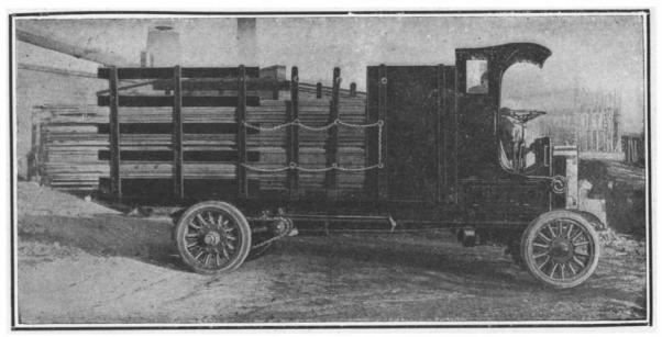
A 5-TON "RAPID" TRUCK AND LOAD OF 63/4 TONS OF HARDWOOD LUMBER AND DRIVER ON SEAT.
