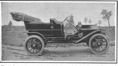
Wheel base, 106 inches; 4 cylinders, 4 x 414 inches; vertical tube radiator; dry battery and high-tension magneto ignition; expanding ring clutch; selective sliding gear transmission; three speeds forward and one reverse; shaft drive.
