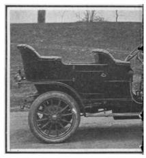
$4\ {\rm cylinders}$  ; water cooled ; make-and-break 'type change gear ; three speeds forw Premier 30-35 horse-
