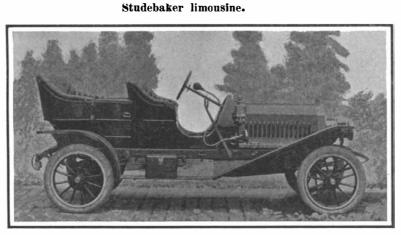
Wheel base, 11014 inches; 28 horse-power; 4 cylinders, 4 x 4 inches; water cooled; jump spark ignition (storage battery); splash lubrication; single silent chain drive inclosed in dust-tight metal case; friction change gear.
