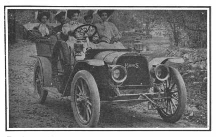
Wheel base, 112 inches; 36 horse-power; 4 cylinders, 4¾ x 5 inches; cellular radiator; dry battery and high-tension ignition; contracting band clutch; selective sliding gear transmission with three speeds forward and one reverse; shaft drive. Haynes touring car.
