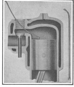
HOW THE CARBON IS SCRAPED FROM THE PISTON HEAD.
