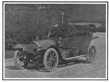
36 horse-power; wheel base, 119 inches; 6 cylinders  $3\frac{15}{15} \times 4\frac{34}{15}$  inches; cellular radiator; storage battery and high-tension ignition; cone clutch; selective sliding gear transmission with four speeds forward and one reverse; shaft drive The Pierce "Arrow."
