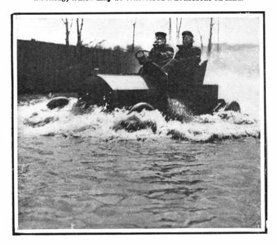
A waterproof Premier car running through water, even though the low-tension magneto is submerged.
