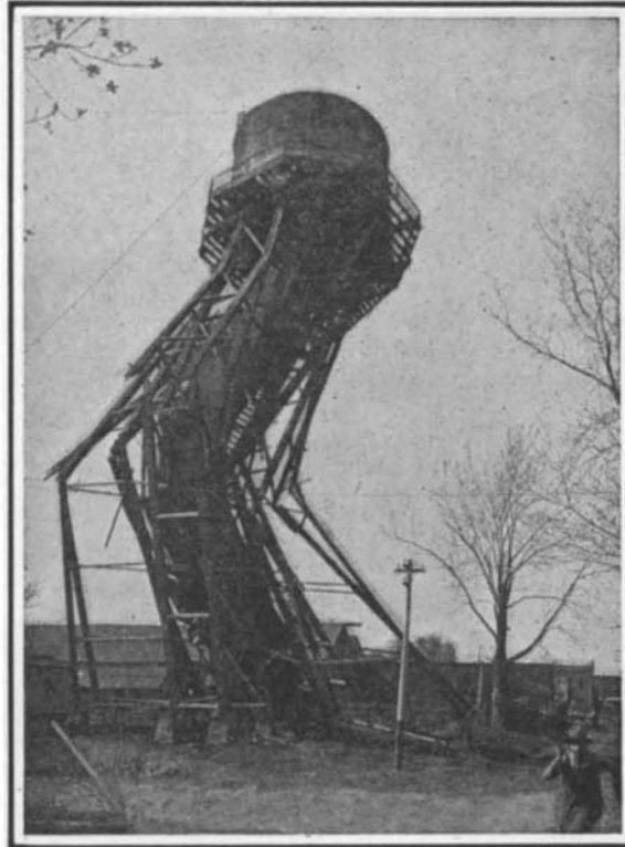
THE DESTRUCTION OF THE WATER TANK AT VERMILLION, S. D.
