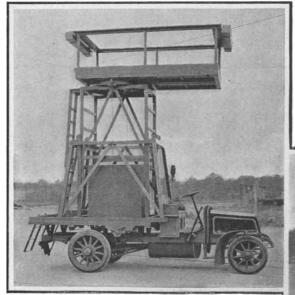
Fig. 1. -- Electrically operated trolley-repairing automobile in service.
