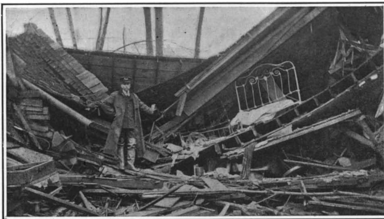
These two houses were carried one block away from their foundations. Two of the occupants perished; five escaped.
