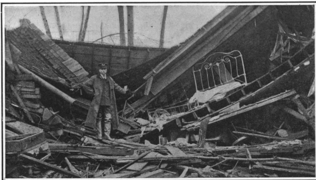
These two houses were carried one block away from their foundations. Two of the occupants perished; five escaped.
