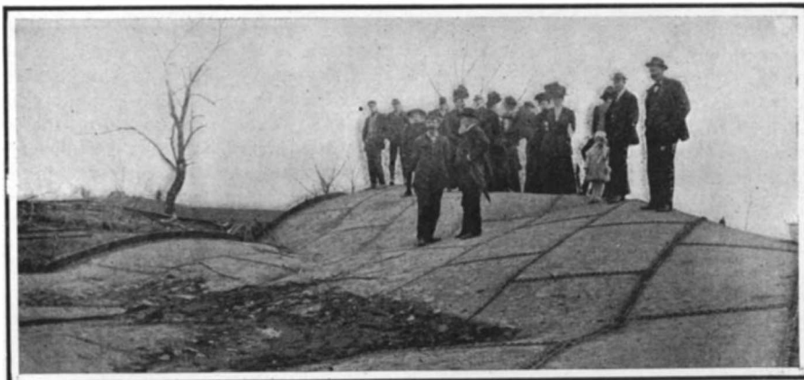
Side of one of the tanks which was found over 100 feet from its foundation.
