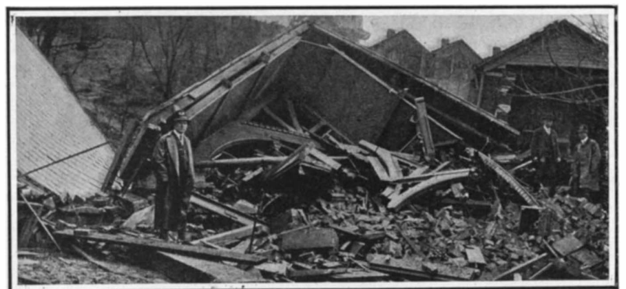
Remnants of the Lutheran church of Parkersburg after the accident.
