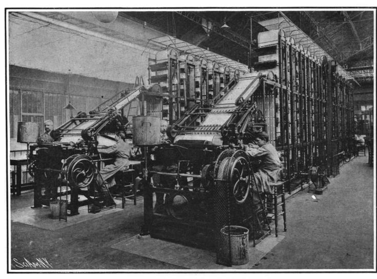
Fig. 1.—Gumming sheets of postage stamps by machine.
