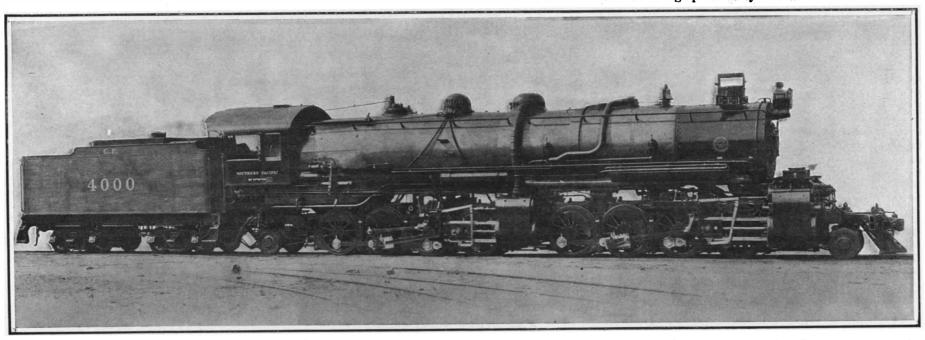
Total weight engine and tender, 300 tons. Drawbar pull, 94,640 pounds, Cylinders: Two high-pressure, 26 inches by 30 inches; two low-pressure, 40 inches by 30 inches Diameter of boiler, 7 feet; heating surface, 6,393 square feet.
