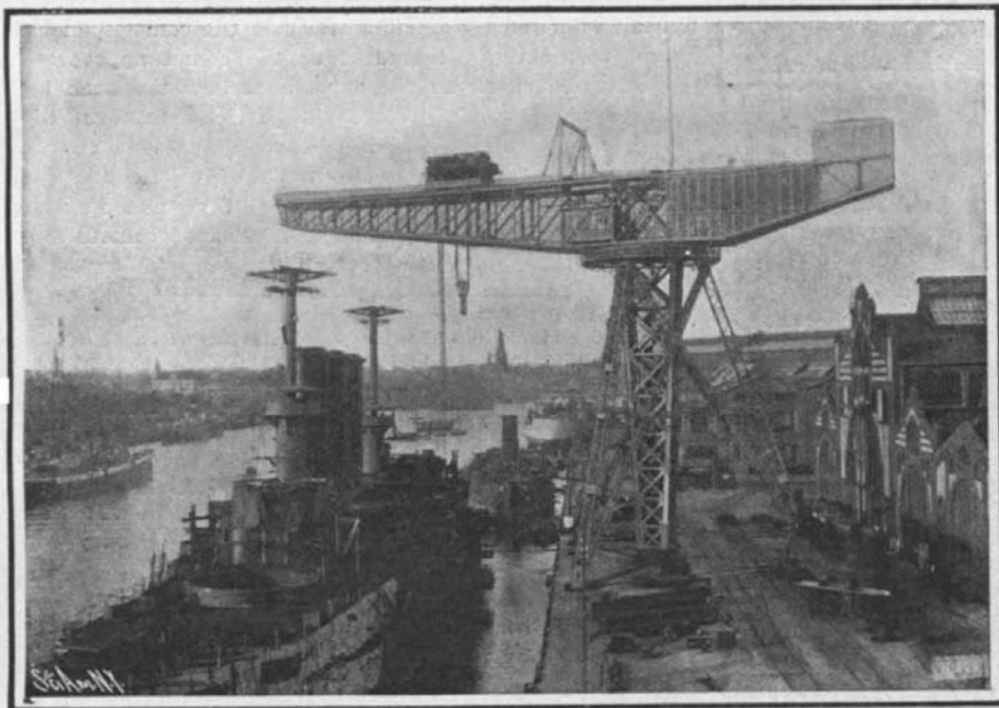
150-ton crane at the Krupp shipbuilding yards at Kiel. Capacity, 45 tons at 125 feet radius and 150 tons at 76 feet radius.
