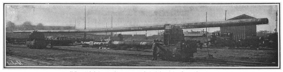
Hollow steel shaft. 17% inches diameter and 150 feet long. forged from 90-ton ingot.
