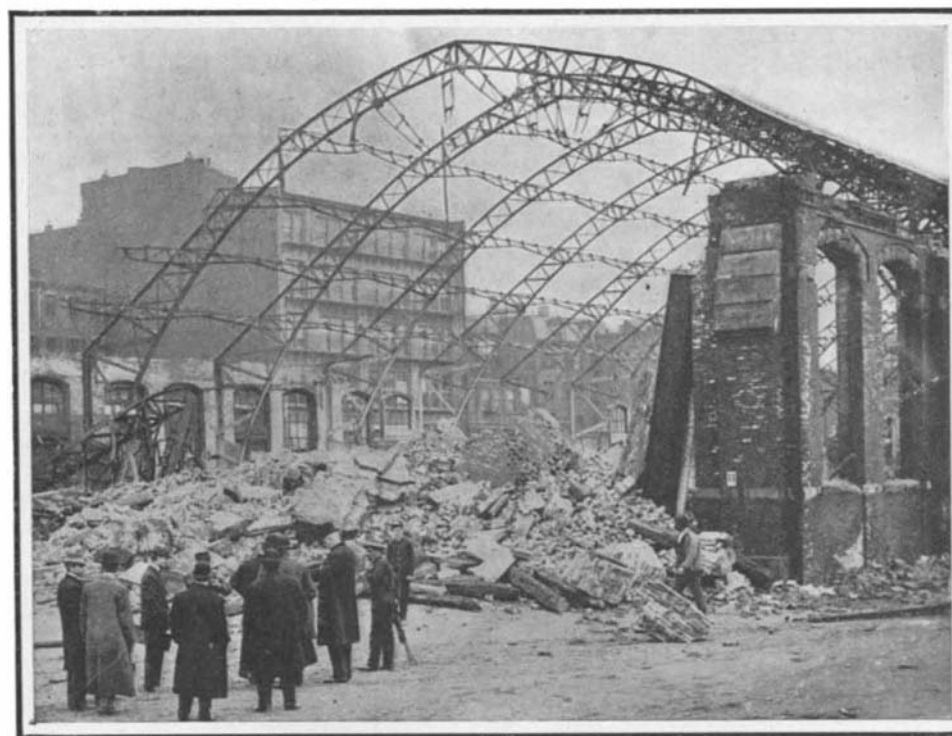
The station after the façade was thrown down.
