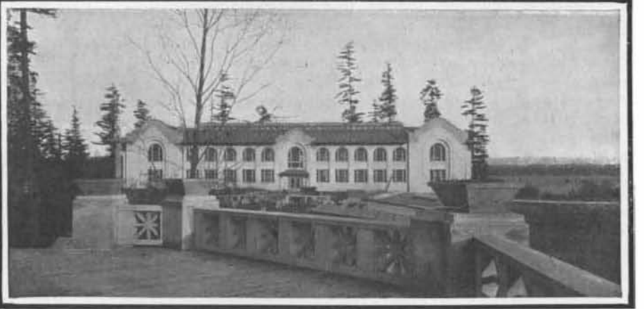
Machinery hall, one of the permanent structures.
