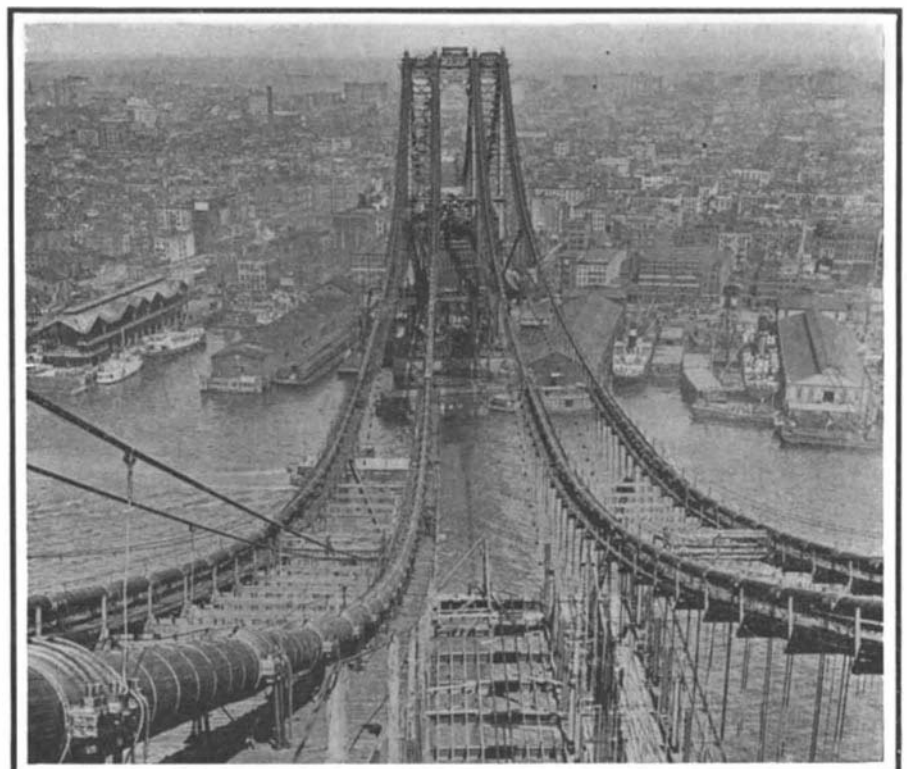
Note on cable to left the saddles which carry the suspender cables. Below is seen the completed portion of the roadway.
