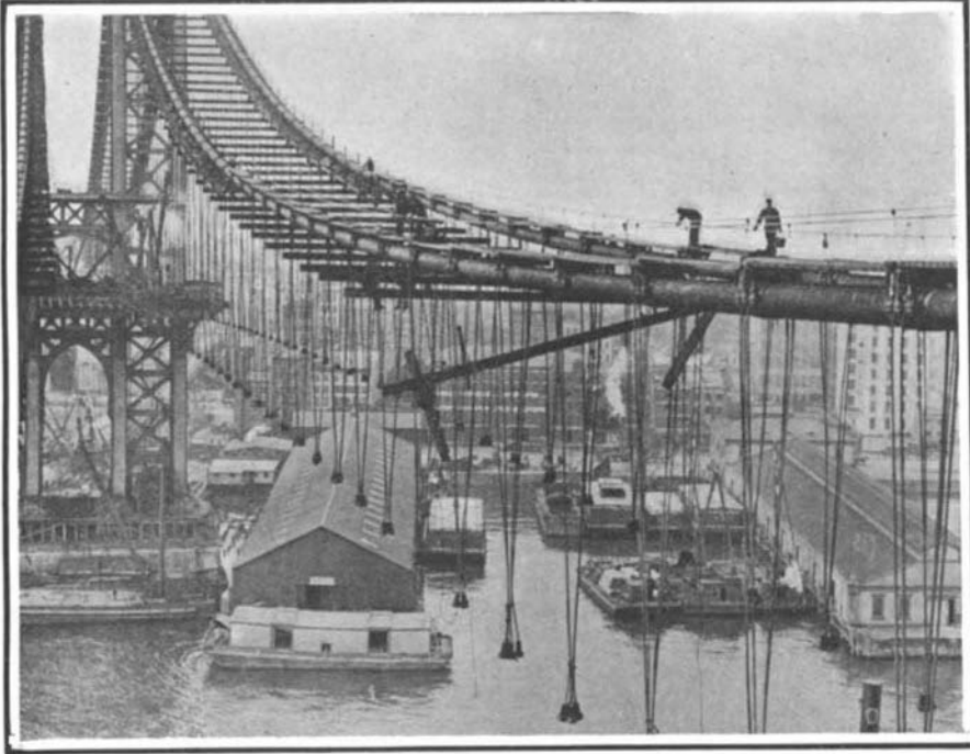
Pair of cables with suspenders in place.
