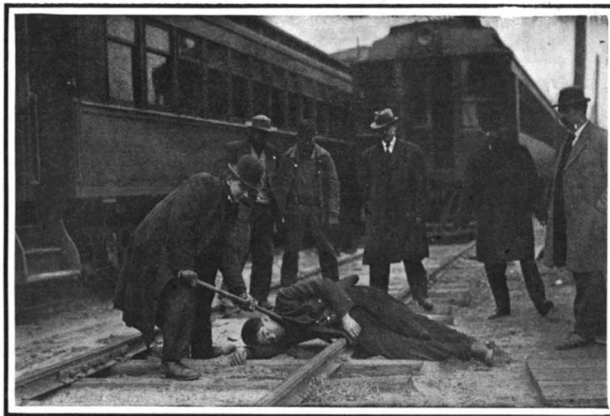
Prying a victim off a live rail with a wooden pole.
